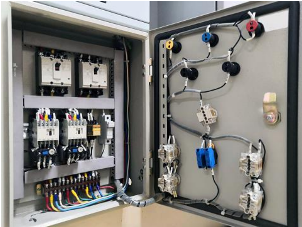
Figure 40: Sample Enclosure Internal Layout
